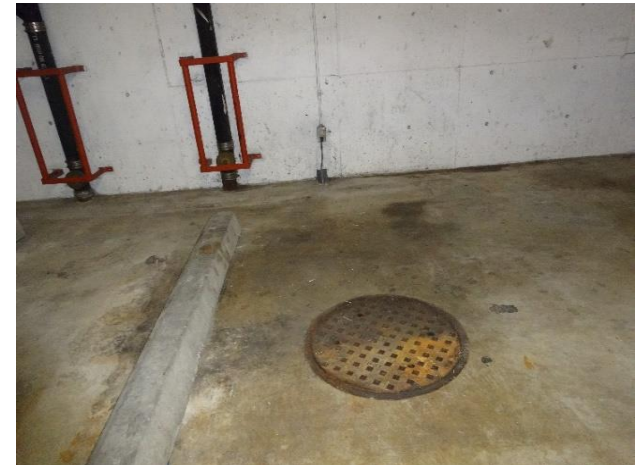
Storm water manhole
