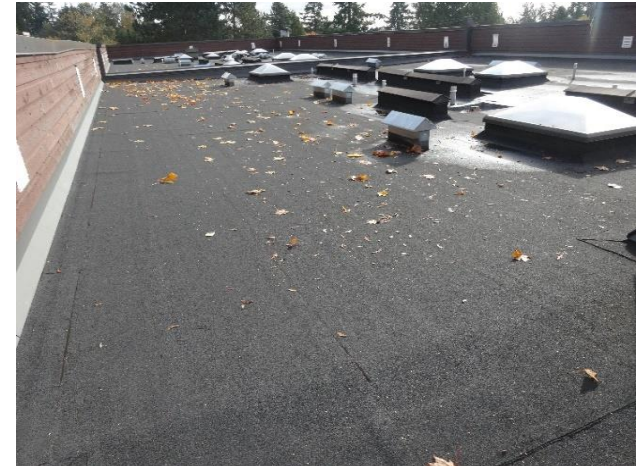
SBS membrane roofing system
