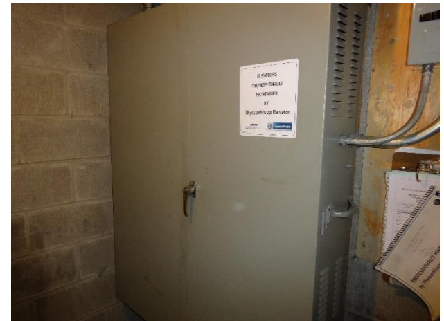
Elevator control panel
