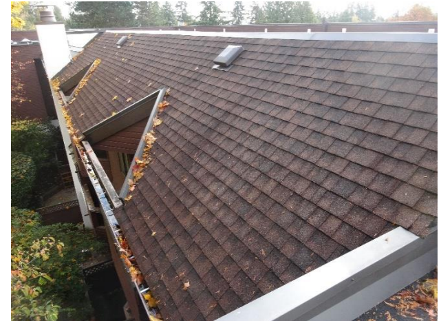
Asphalt shingle roofing system
