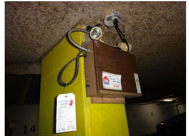
Obsolete emergency lights and battery package
