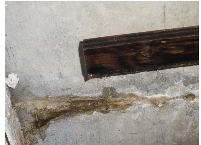
Leaking crack on suspended slab
