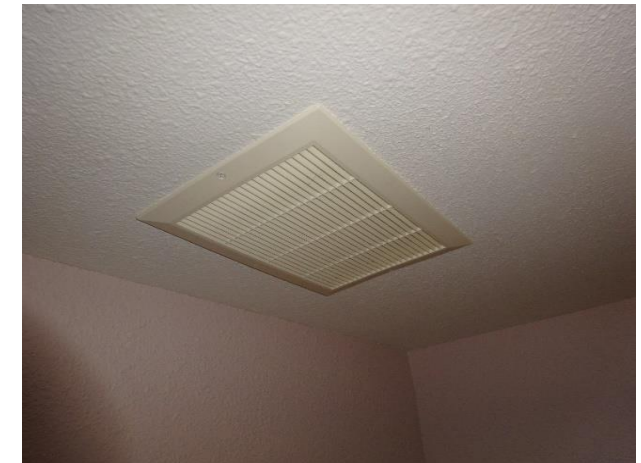
Exhaust fan in washroom
