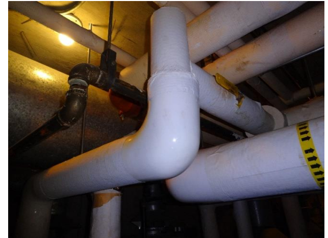
Hot water heating piping and valves
