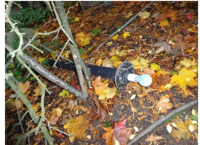
Fallen post with light fixture
