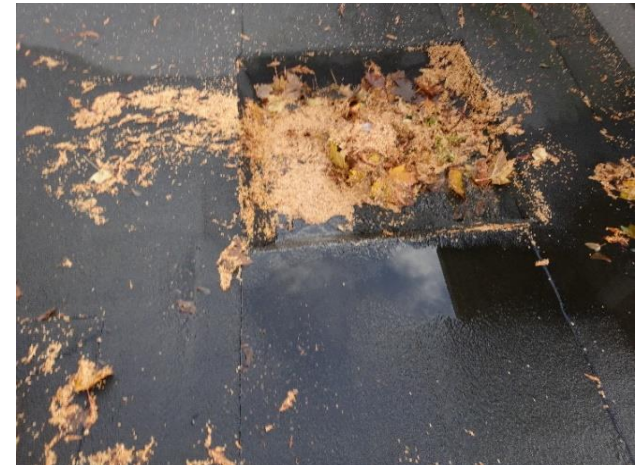
Clogged roof drain
