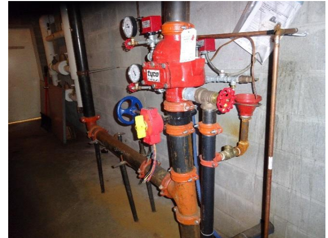
Distribution station and control valve
