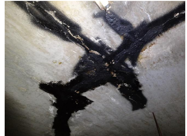
Repaired crack on the suspended slab but still leaking
