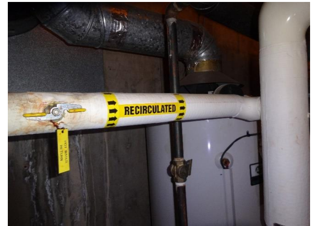
Domestic hot water piping and valves
