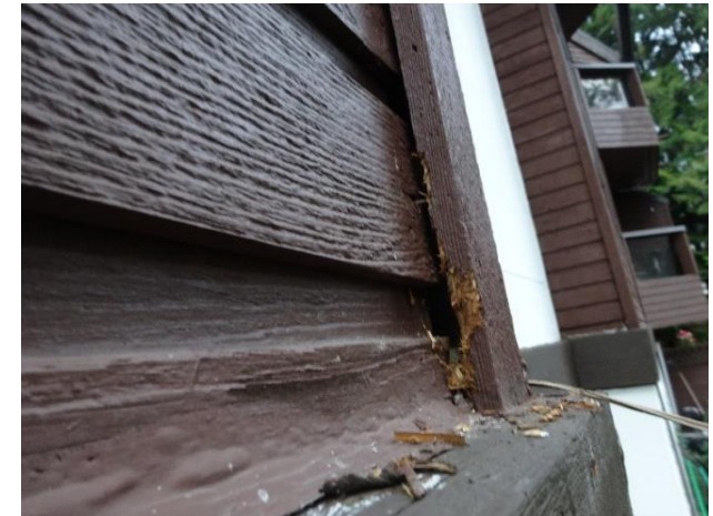
Rotten wood cladding/trim
